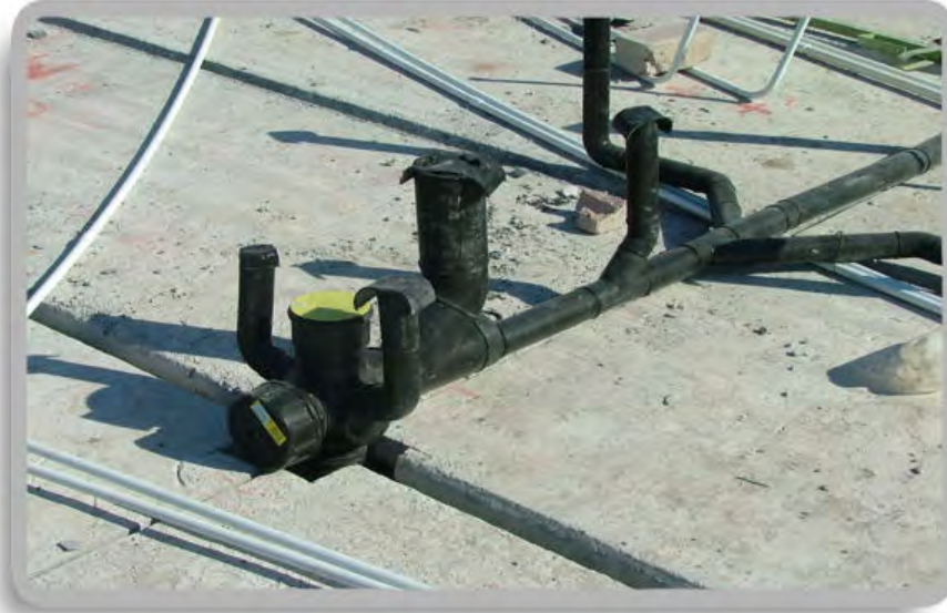
Plumbing and electrical conduits placed prior to screeding. Conduits should be run over the top of the Topfloor slab.
