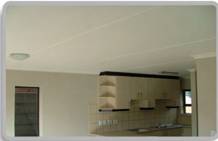
"V" joints on the soffit are a feature of Topfloor Hollow-Core slabs and should not be plastered closed.
